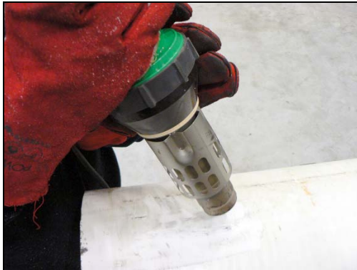
Heat the tip of the PP-Meltstick with the hot air tool.
