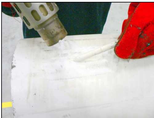
Apply the molten material of the PP-Meltstick into the damaged area by turning the stick.
