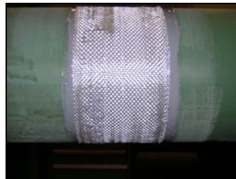
Circumferential damage repair / S1401 epoxy application and thickness measuring / 18 mils to 20 mils.
