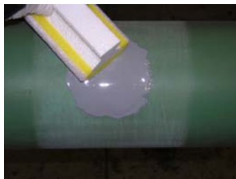
Local scratch repair / S1401 epoxy application and thickness measuring / 18 mils to 20 mils.
