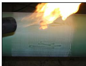
Preheating and temperature measuring / 50°C to 60°C
