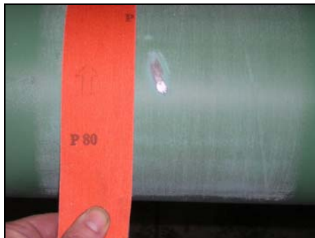
Roughening of FBE line coating with P80 abrasive paper.
