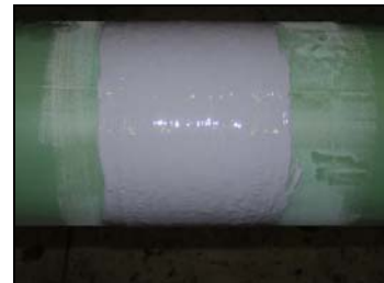
Circumferential damage repair / S1401 epoxy application and thickness measuring / 18 mils to 20 mils.
