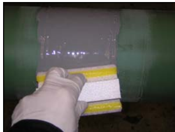
Circumferential damage repair / S1401 epoxy application and thickness measuring / 18 mils to 20 mils.
