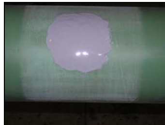
Local scratch repair / S1401 epoxy application and thickness measuring / 18 mils to 20 mils.
