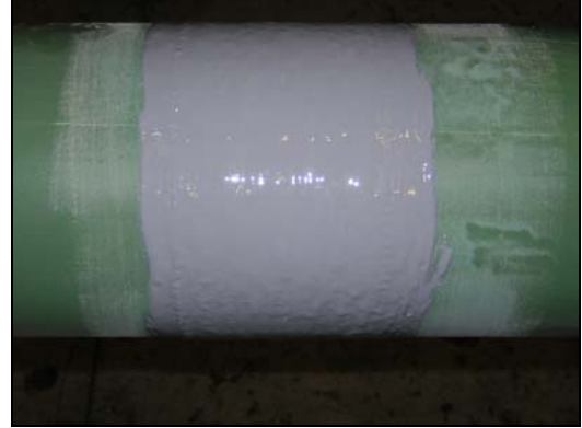
Finished S1401 repair of scratch in FBE line coating.
